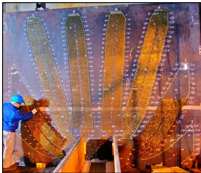
Figure 4: CP2 condenser tubesheet 3
